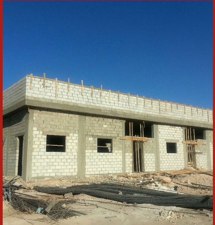
Under construction: workers' center in Al-Hassan Industrial Zone
