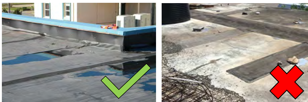
Figure 7-1: Good vs. Poor Insulation of Roof Slab
