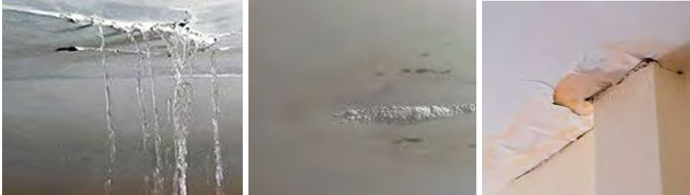
Figure 7-4: Common leakage problems
